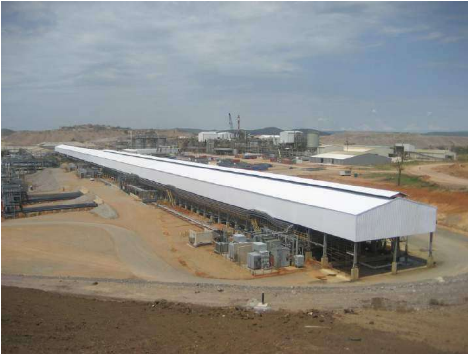
Figure 1-3 Tankhouse Completed as seen in November 2013
