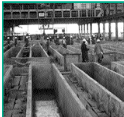
(right) A rebuilt mill sump is lowered into place
