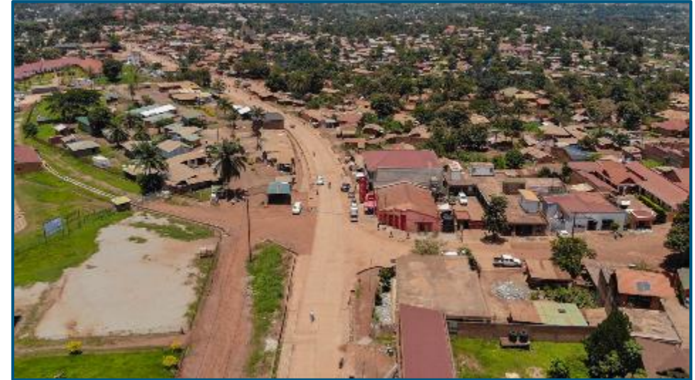
Construction of concrete road in Durba
