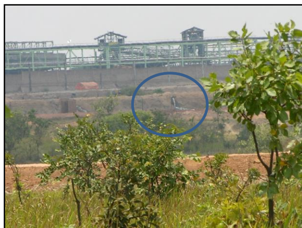
KCC plant waste (October 2013)
