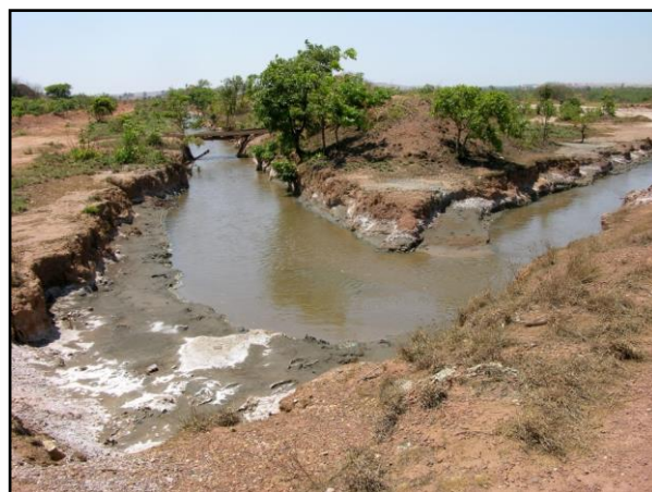
Bend in the Albert Canal, where it has been diverted (October 2013)
